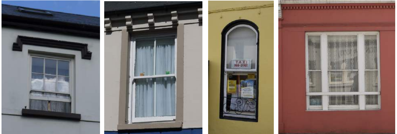
Church Street retains few early sash windows. Window replacement is one of the most frequent alterations that detracts from the traditional character. Every effort should be made to repair and retain surviving early windows as above. Left to right: 35, 46, 55, 93 Church Street.
