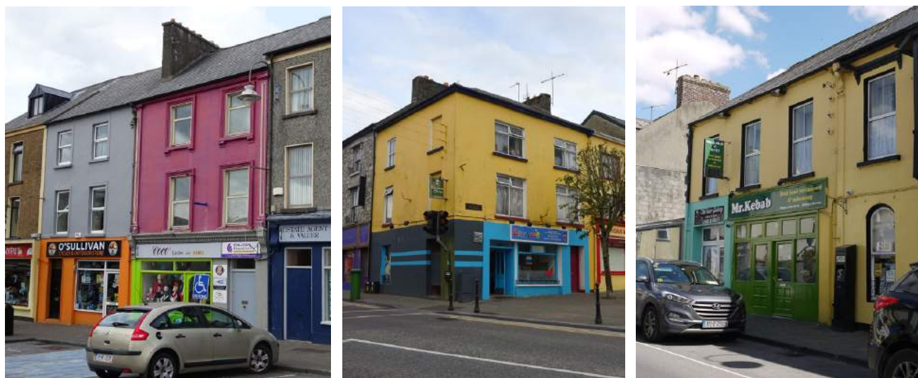
Examples of how a lack of coordination between ground and upper floor paint colours detracts from the overall composition of the entire facade.
