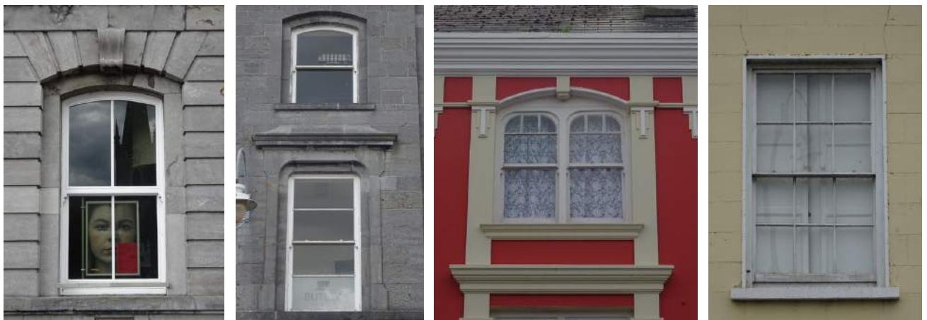
Samples of early sash windows in the The Square. Left to right: 8, 12 19, 36 The Square.
