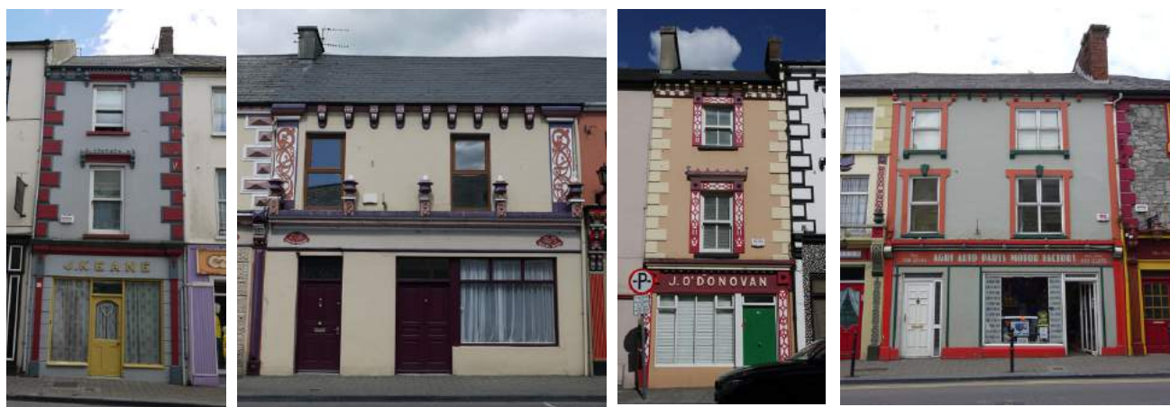
Examples how how a paint colours can unify the shopfront and upper floors, enhancing the streetscape.
