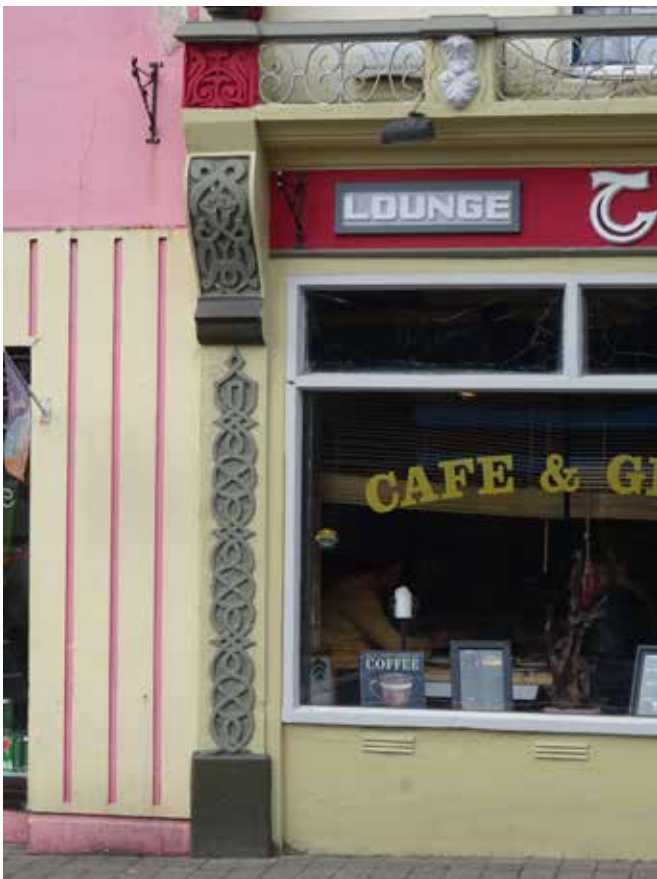
12MST_07 Detail of shopfront
