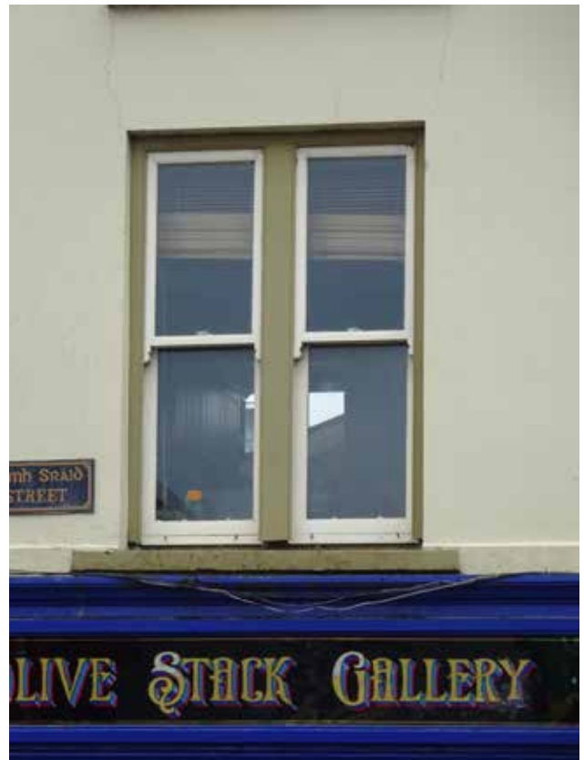
04MST_04 Second floor window
