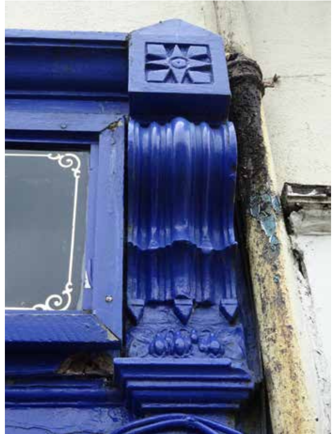
04MST_08 Detail of shopfront
