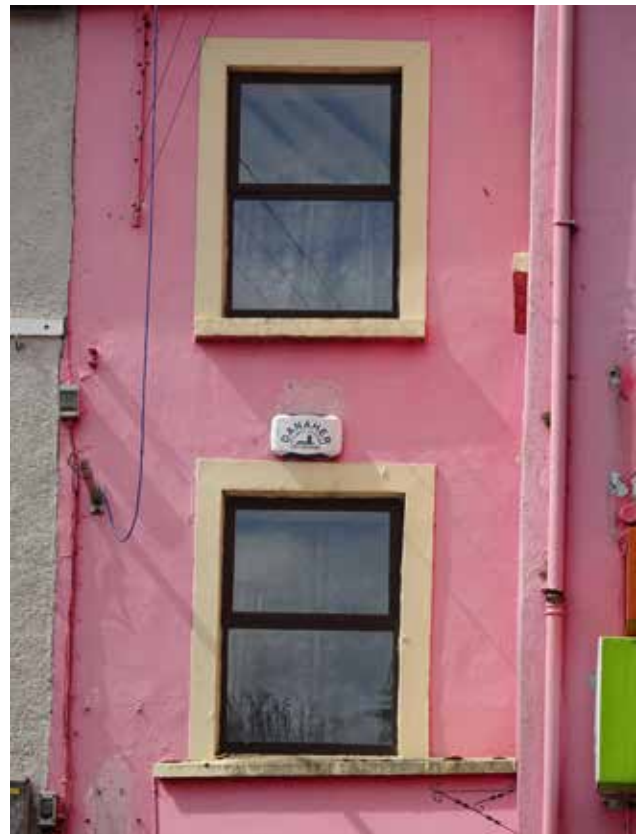
11MST_04 First and second floor windows
