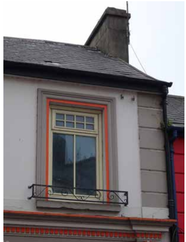
18MST_02 Detail of chimneystack, roof and first floor window
