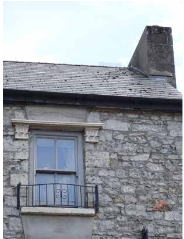
10MST_02 Detail of roof, chimneystack and second floor window
