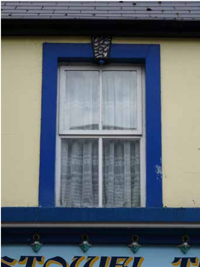
15MST_03 First floor window
