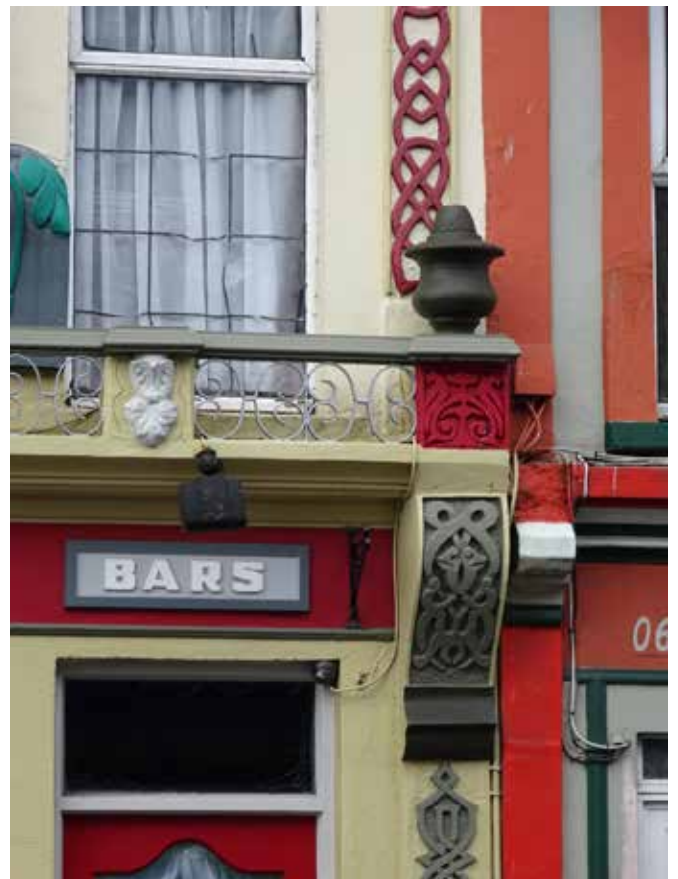
12MST_08 Detail of shopfront
