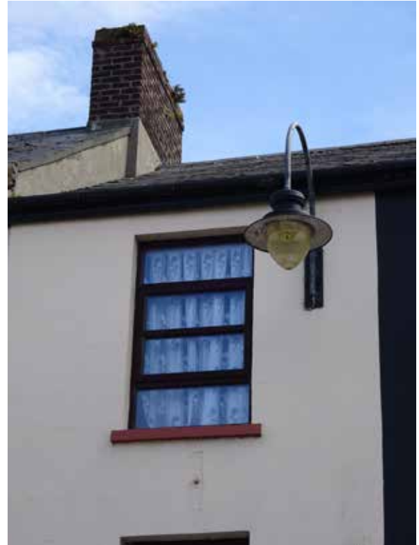
07MST_02 Detail of roof, chimneystack and second window
