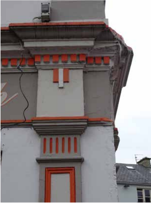
18MST_05 Detail of shopfront
