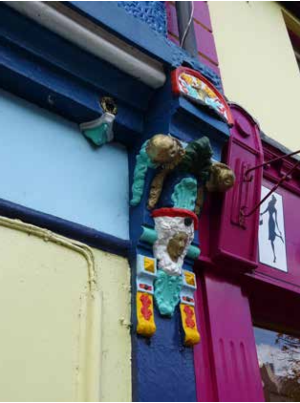
15MST_09 Detail of shopfront
