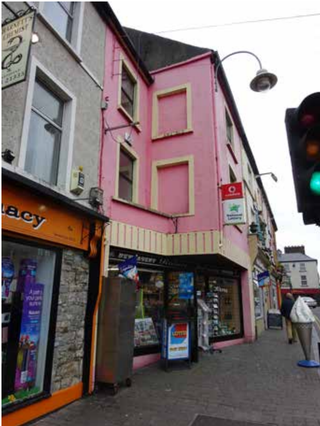
11MST_03 West-facing portion of front elevation
