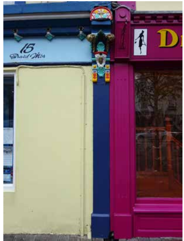
15MST_06 Detail of shopfront
