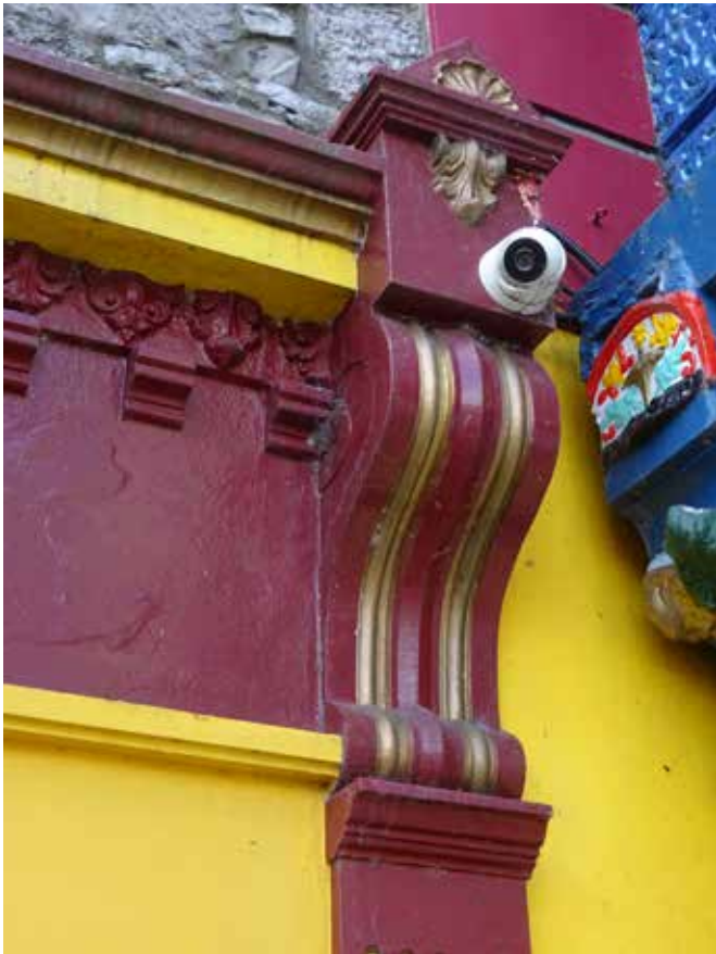
14MST_07 Detail of shopfront
