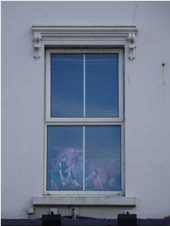
06MST_03 First floor window
