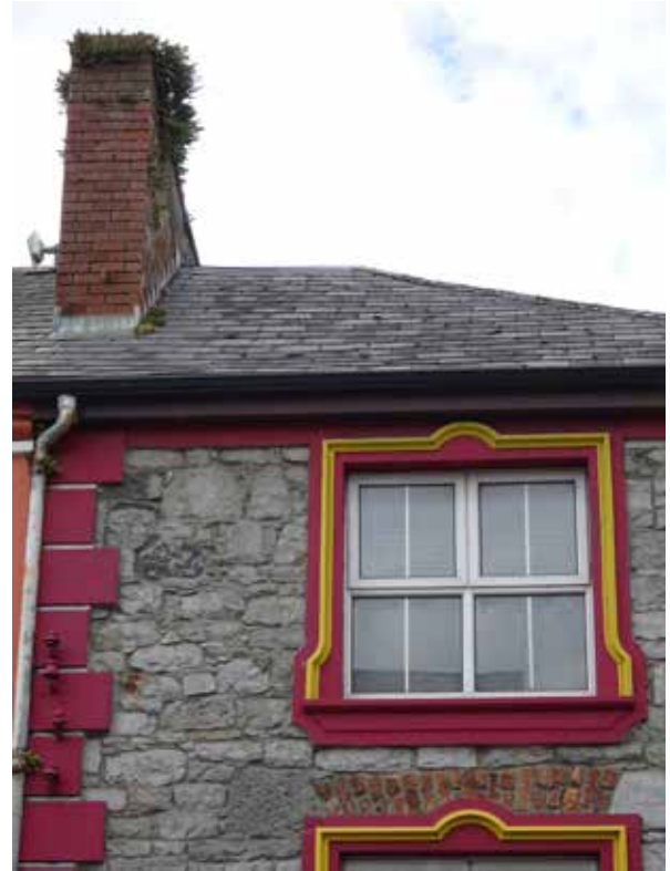
14MST_02 Detail of chimney stack, roof and second floor window
