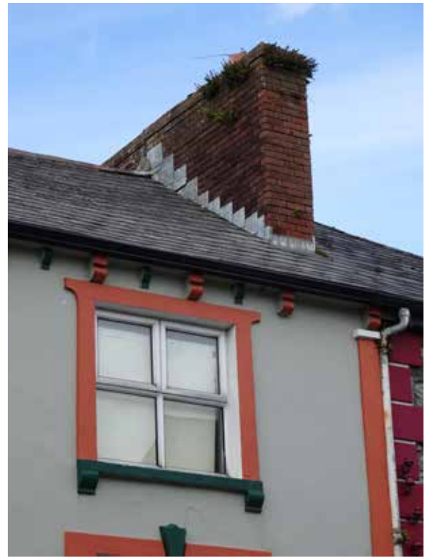
13MST_02 Detail of roof, chimneystack and second floor window
