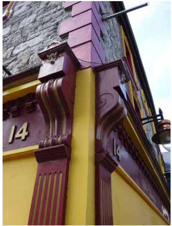
14MST_06 Detail of shopfront
