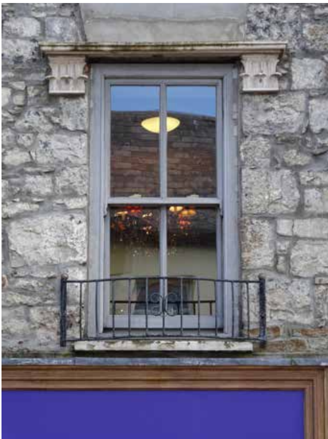
10MST_03 First floor window
