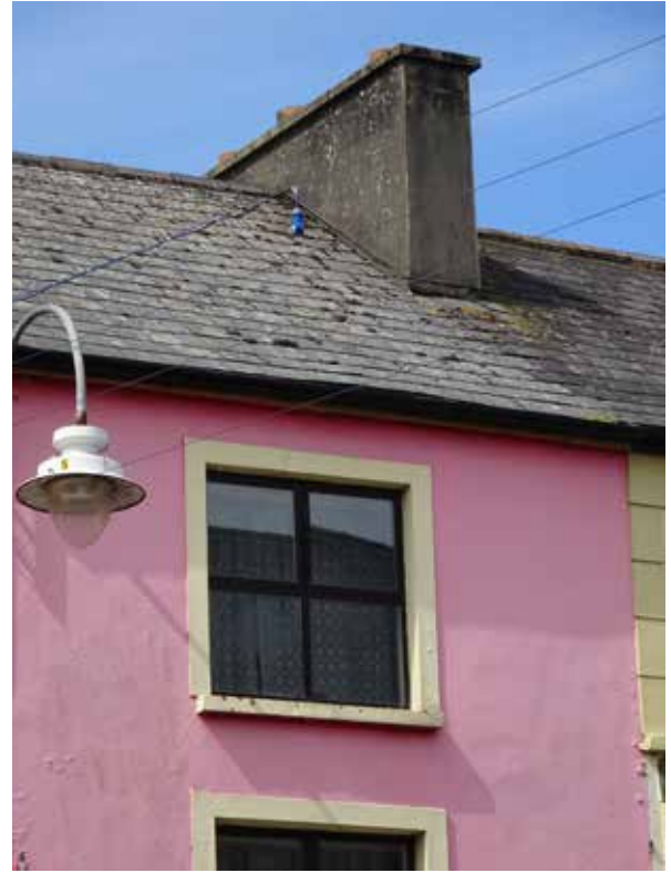
11MST_02 Detail of roof, chimneystack and second floor window
