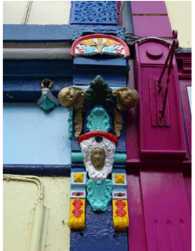
15MST_08 Detail of shopfront
