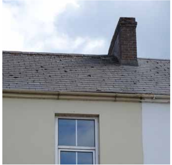
05MST_02 Detail of roof and chimneystack
