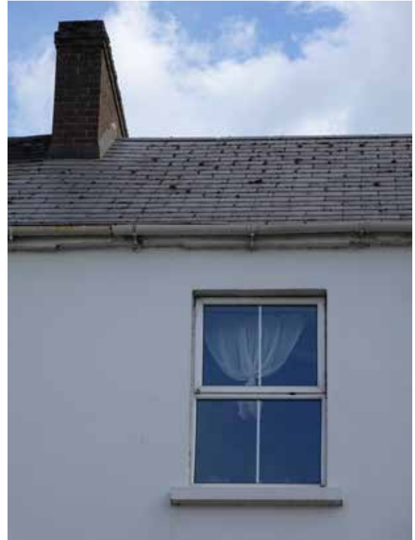
06MST_02 Detail of roof and second floor window
