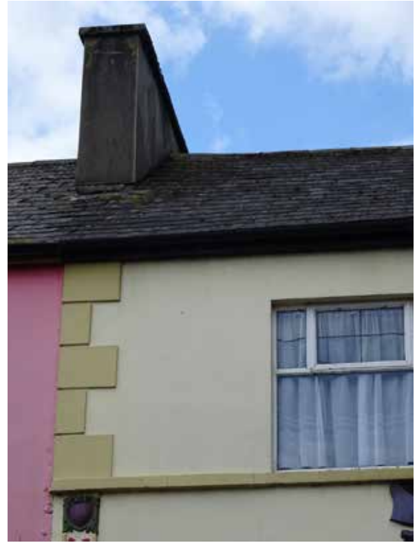
12MST_02 Detail of roof, chimneystack and second floor render
